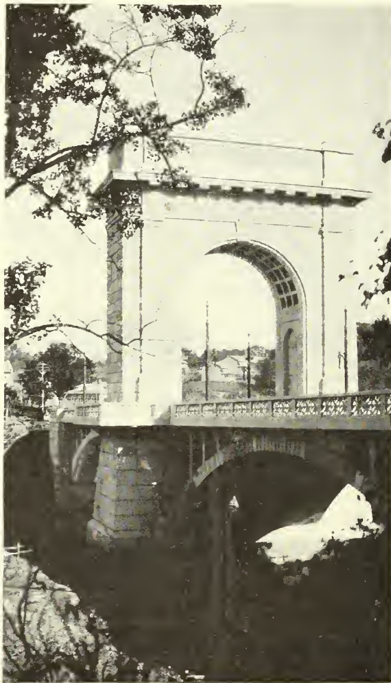
Posts of Delaware County, Pennsylvania, helped dedicate this concrete memorial bridge over Plum Creek which bears bronze tablets recording the names of the county's World War dead.
